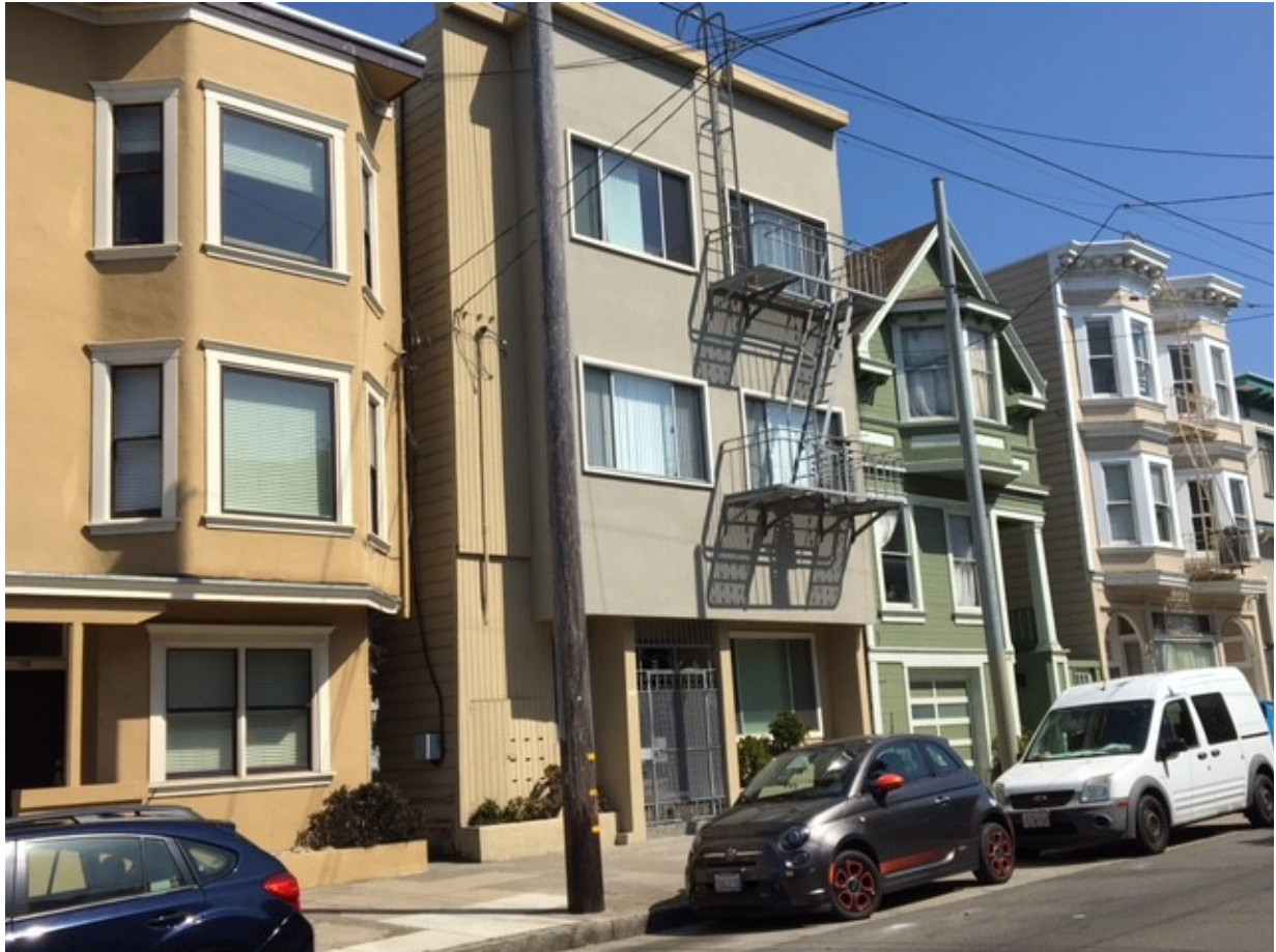
Figure 4. Some of the “Richmond Specials” that replaced Victorian single-family homes
