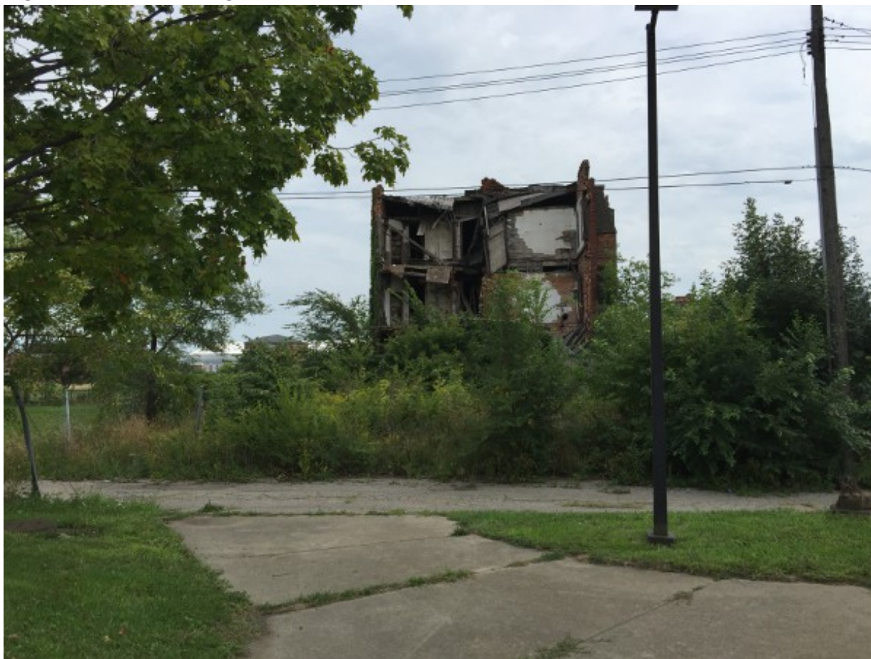
Figure 1. Derelict housing in Cleveland, Ohio
